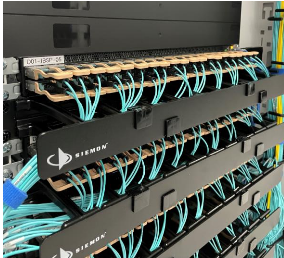
MTP Jumpers into Leaf Switches
